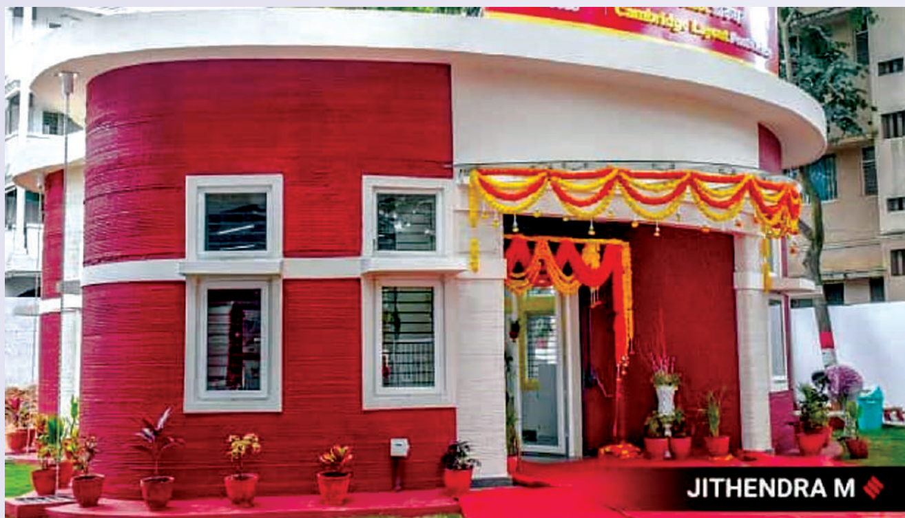
India's first 3D-printed post office located in Bengaluru's Cambridge Layout. (Express photo by Jithendra M)
