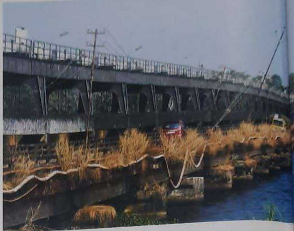
THE THANNEERMUKKOM BUND , a barrier constructed in 1974 to prevent saltwater intrusion into the Kuttanad lowlands.
